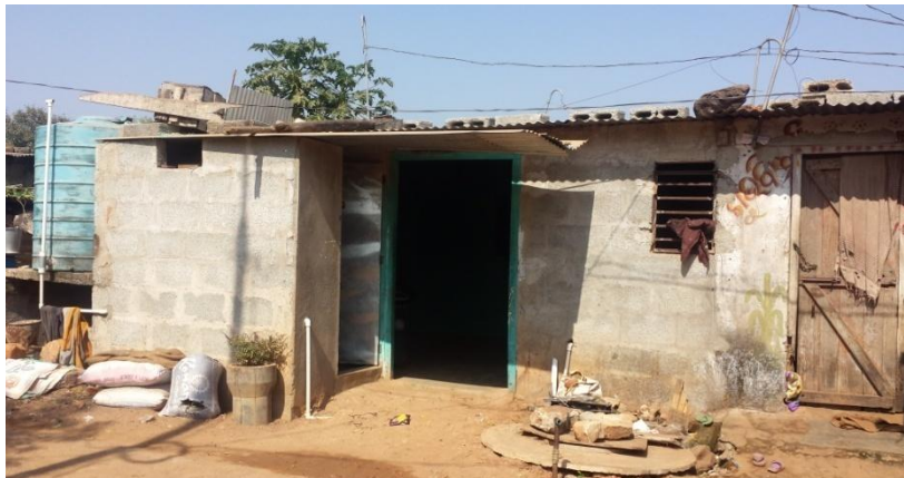
Toilet connected to sewer line in Sitanath Nagar , Bhubaneswar
