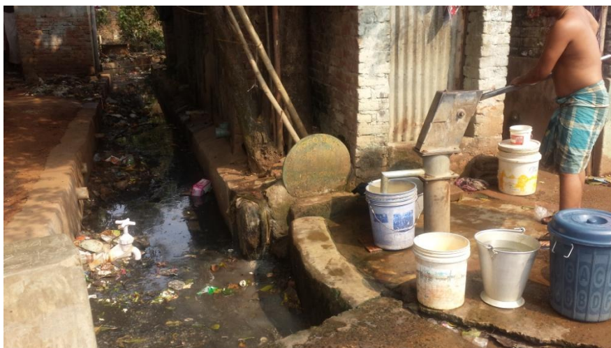
Photograph shows how water source, toilet and drainage disposal are adjacent to each other-encouraging contamination in Shantipalli , Bhubaneswar
